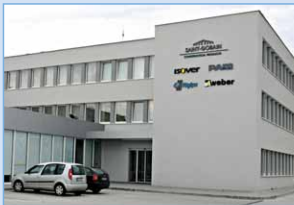
Sídlo firmy Saint-Gobain Construction Products, Bratislava
